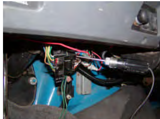
Figure 7. Locate and determine the wires needed. A wiring diagram and/or test light will be helpful.
