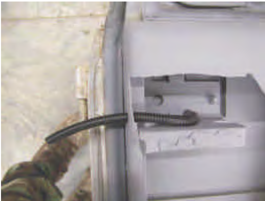
Figure 4. This cut-away of a door shows the required location of the second hole. It was necessary to locate the hole nearer the inside of the door to avoid hitting the lower section of the window channel. The wire loom shows the desired wire routing.
